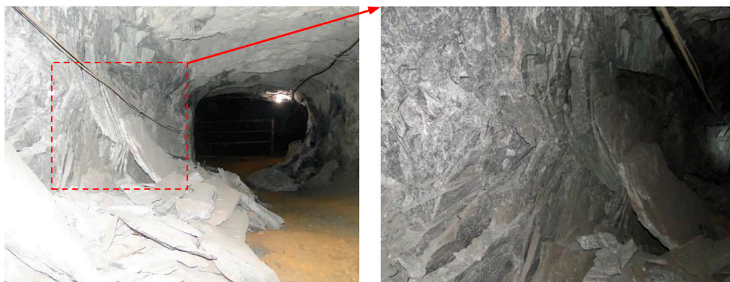
FIGURE 2 Spalling failure of the ramp surrounding rock in the 13# stope.
