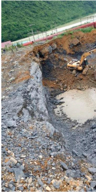
FIGURE 7 | Main rock blasting of reserved rock wall.
