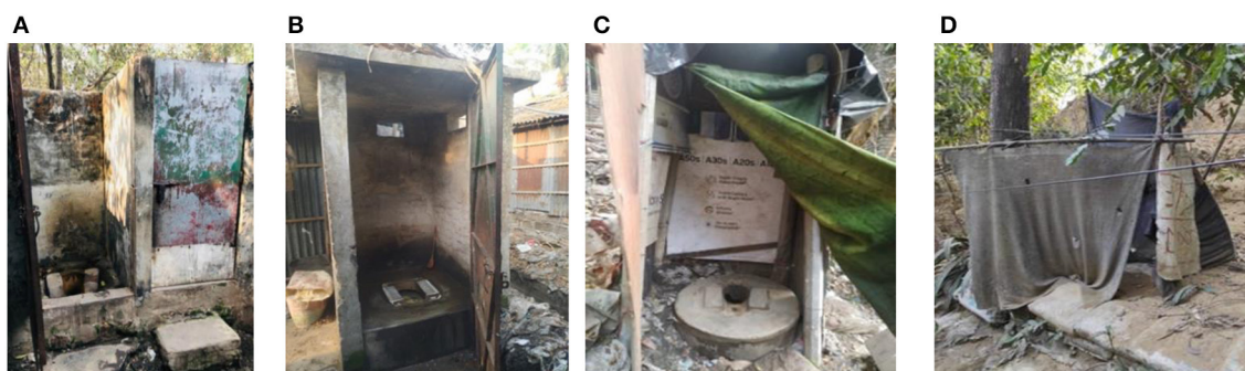
FIGURE 2 Toilet facilities in slum areas. (A) Pit latrine without slab, (B) pit latrine with slab, (C) hanging toilets, (D) open field toilet.
