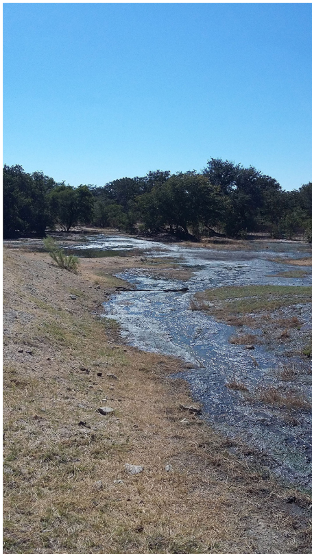
FIGURE 2 Overflowing of untreated wastewater from a Waste Stabilization Pond (WSP) in Eenhana municipality in 2018. Photo: Fanny Frick-Trzebitzky.
