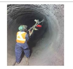
FIGURE 3 | SAPL method used for large conduits. https://www.vectorconstruction.com/geospray-pipe-and-culvert-lining.
