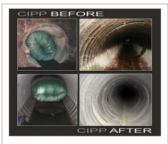
FIGURE 5 | CIPP before, during, and after installation. https://www.prweb.com/releases/uspipeliningpressrelease/june2016/prweb13466103.htm.
