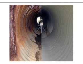
FIGURE 2 | Machine pipe renewal for SAPL. https://www.estormwater.com/ pipe-distribution/pipeline-rehabilitation-products.
