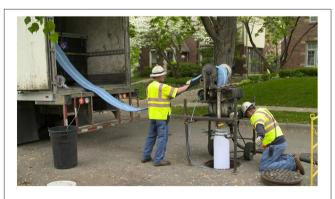
FIGURE 4 | Equipment used during the installation of CIPP. https://www.aegion.com/capabilities/cured-in-place-pipe/insituform-cipp.
