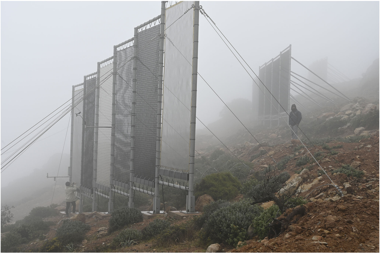
PHOTO 1 | Fog water collection systems (Credit: Aqualonis).
