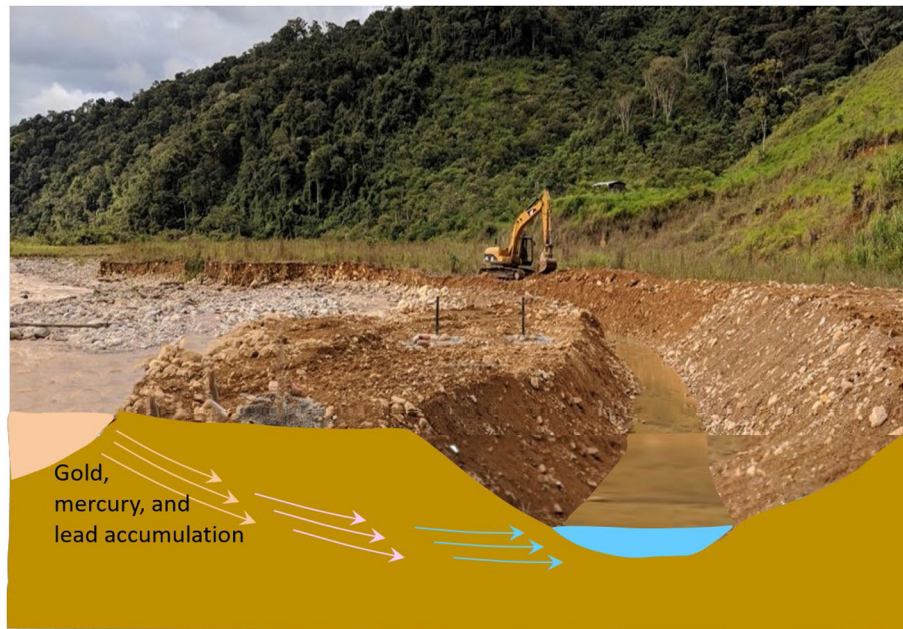
GRAPHICAL ABSTRACT | Completed lateral channel oriented parallel to flow (away from camera). Rio Nambija forms the left boundary of the gravel bar, the lateral channel forms the right boundary.
