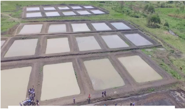
Plate 4 | Siunga Aquapark in Butula Sub-county.
