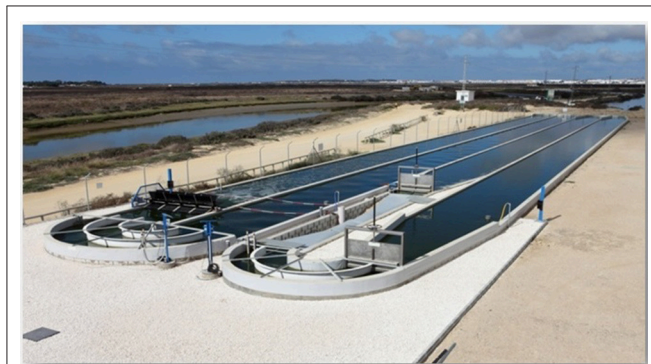
FIGURE 3 | Image of raceway reactors operated by FCC Aqualia in ALLGAS project for wastewater treatment and nutrients recovery using microalgae. Left, a regular raceway reactor, Right, the LEAR system.
