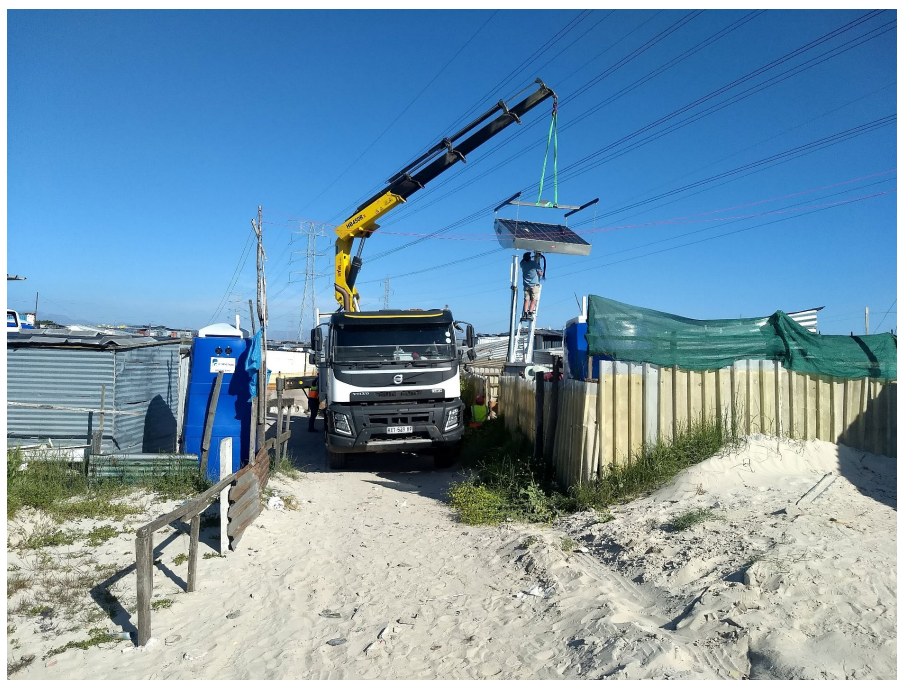
FIGURE 2 Installation of the microgrids (source: Authors).
