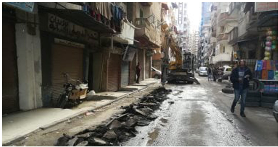
FIGURE 8 Streets of Elmandara Qebly area that have poor maintenance. Source: Author.
