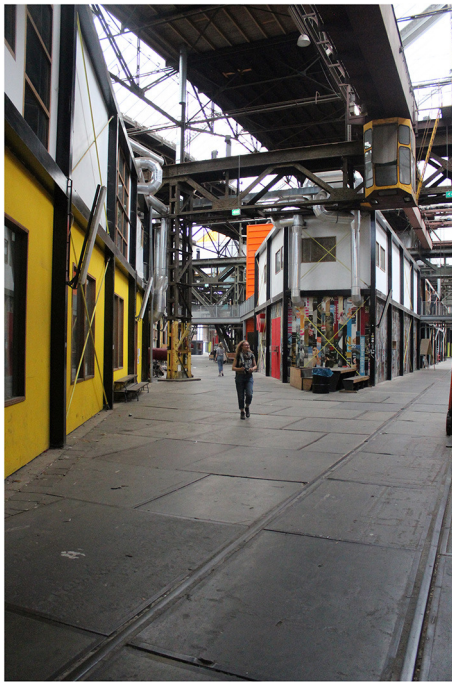
FIGURE 6 Two-story supporting structure with ateliers inside the Shipbuilding Warehouse at NDSM Wharf (photograph by Shuguang Zou).
