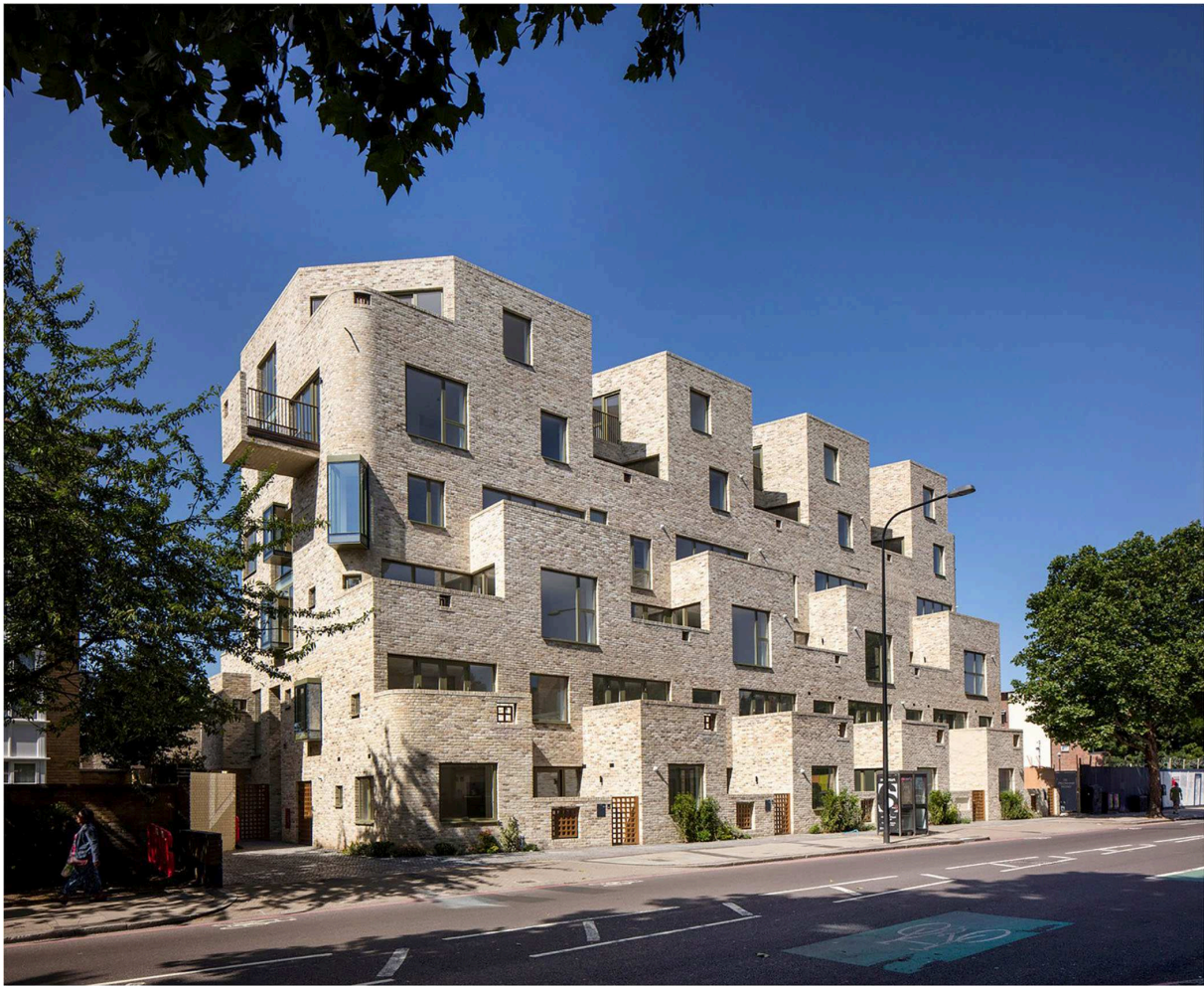
FIGURE 2 View of front elevation from Peckham Road (Ravenscroft, 2020).
