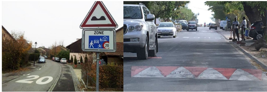
FIGURE 1 | Traffic calming: Narrowed lane and speed humps for a 20 km/h limit on a residential road in Switzerland, and speed tables either side of a pedestrian crossing in Senegal (Source: photos by the author).
