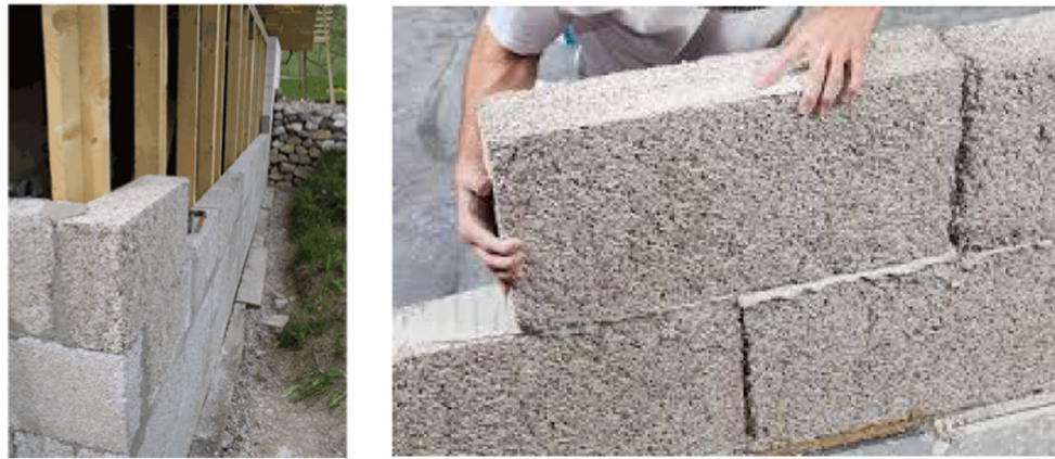
FIGURE 2 Typical example of precast Hempcrete Block Building Construction (Left, Courtesy of Wikipedia, https://en.wikipedia.org/wiki/Hempcrete ; Right, https://www.iso hemp.com/en/hemp-blocks-buildings-hempro-system ).
