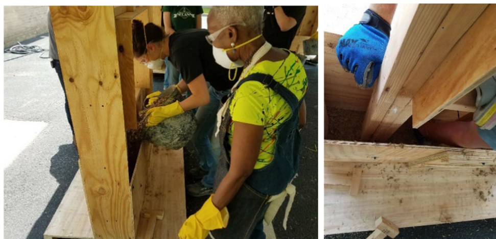
FIGURE 7 Hempcrete cast-in-place demonstration by Americhanvre Inc.
