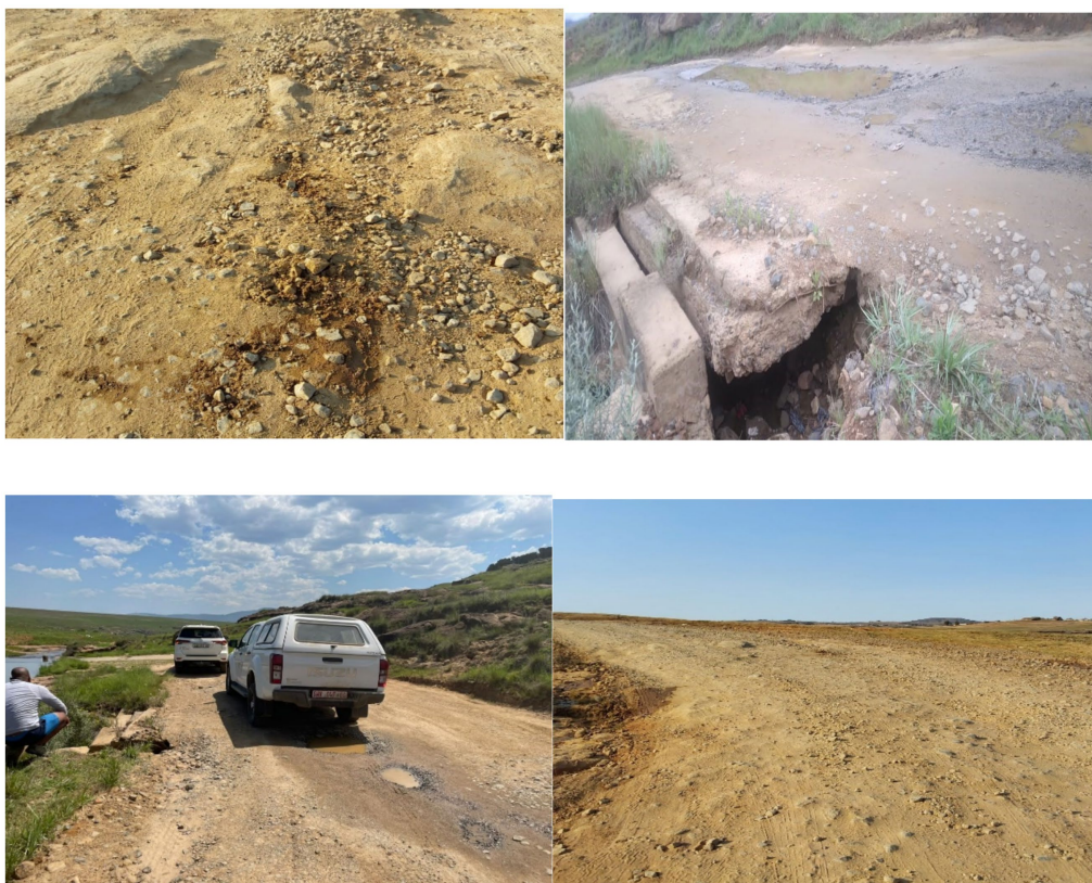
FIGURE 1 Examples of poor road conditions from Mdeni to Upper Tsitsana. Source: Author's camera.
