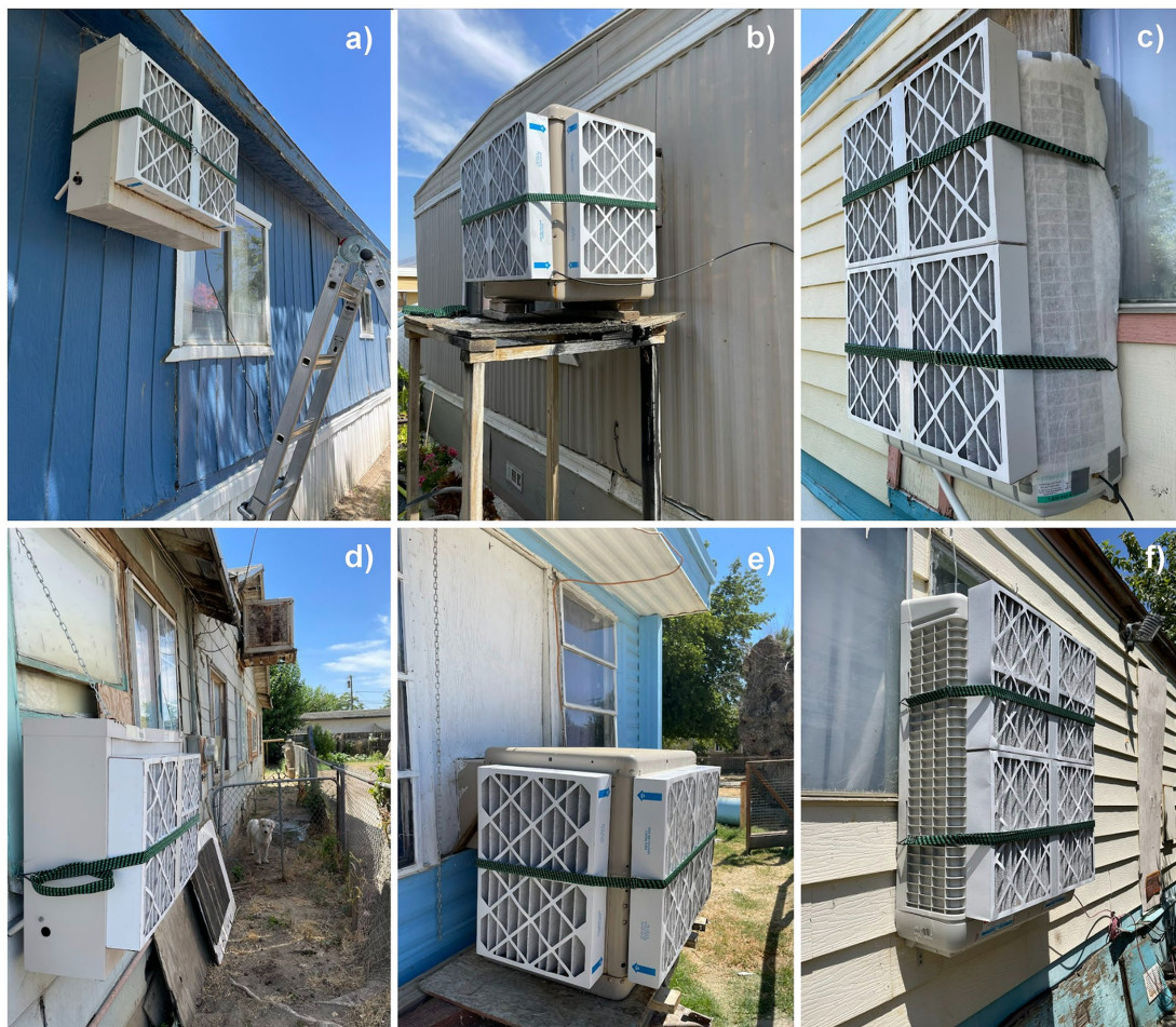
FIGURE 2 Evaporative Coolers in the study region with our DIY Filter Interventions: (a, d) are single intake ECs, (b, e) are 3 side intake ECs, (c, f) are curved side intake ECs in which (f) already had the sides blocked and for (c) we used a hybrid solution of Sheet Filter media with our DIY Filter solution.
