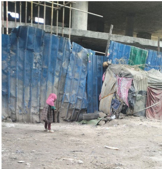
FIGURE 18 Safety risks for children. Addis Ababa, Ethiopia, December 2023. A little girl is standing next to her shelter (Shera Bet), the type of shelter homeless people live in. There is a risk of stones being thrown at the shelter if construction is built above it. This could endanger the girl's safety. Sadly, officials often destroy the shelter without prior warning, leaving the family with nothing to live on. I took a photograph of the shelter to represent my living situation (Image and quote credited to a 28-year-old mother experiencing street homelessness).
