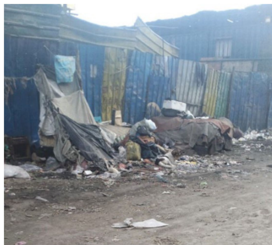
FIGURE 11 A mothers' shelter is demolished. Addis Ababa, Ethiopia, December 2023. My home is constantly being torn down, so it is difficult to say anything about it. I mean, um... I am not interested in discussing this matter. My daughter's friends brought us clothing in yellow plastic bags last time (Her eyes welled with tears). As our shelter was demolished, we burnt everything that remained (Image and quote credited to a 28-year-old homeless mother of three children).
