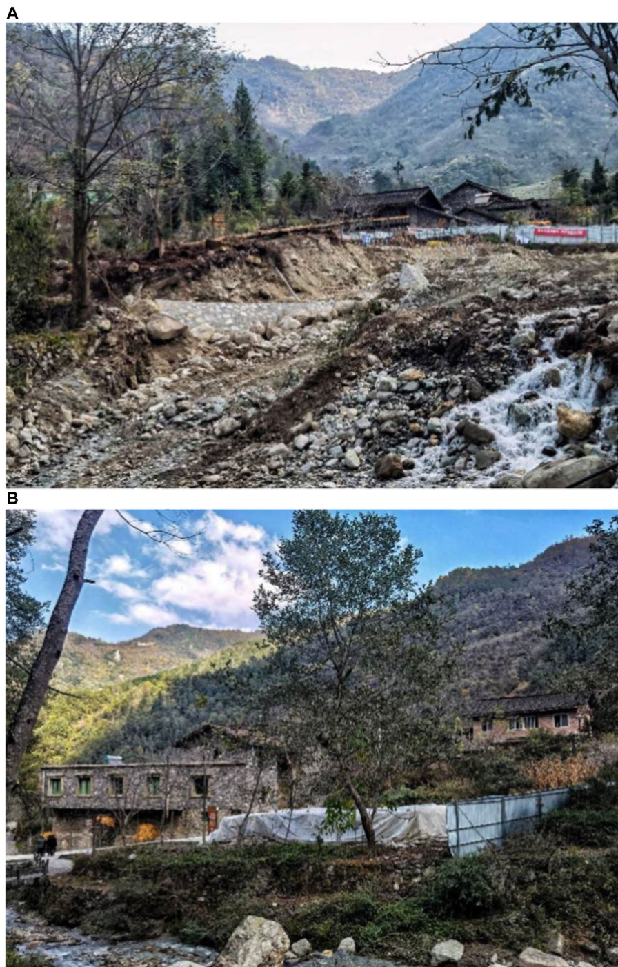
FIGURE 6 Post-disaster situation by the “9.5” Luding Earthquake in Xieluo-buzi village (Source. Photographed by the author): (A) Physical environment damaged by the “9.5” Luding Earthquake in Xieluo-buzi village; (B) Road and environment damaged by the “9.5” Luding Earthquake in Xieluo-buzi village.
