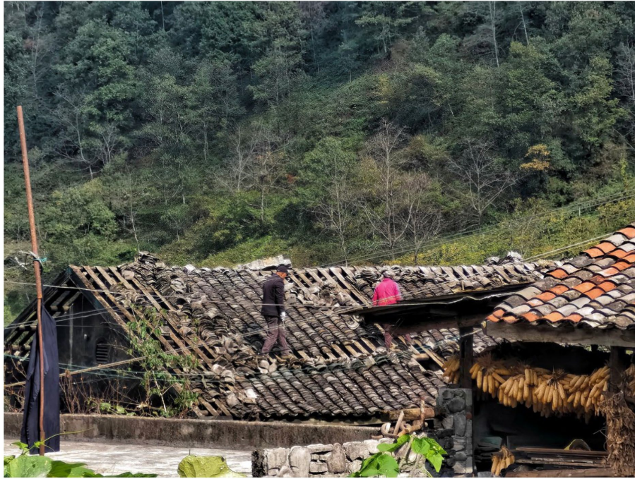
FIGURE 4 Traditional houses damaged by the "9.5" Luding Earthquake in Xiluo-buzi village (Photographed by the author).
