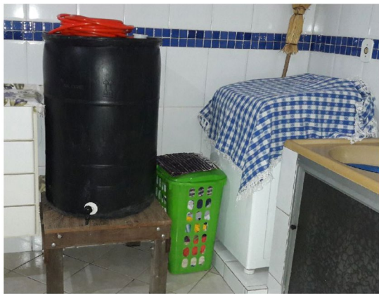
FIGURE 2 Arrangements made by participant Mônica at home; the installation of a container to collect and reuse water drained from the washing machine.
