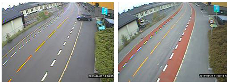
FIGURE 1 | Camera capture at Kongsveien before and after the cycle lane was recoated with red asphalt.
