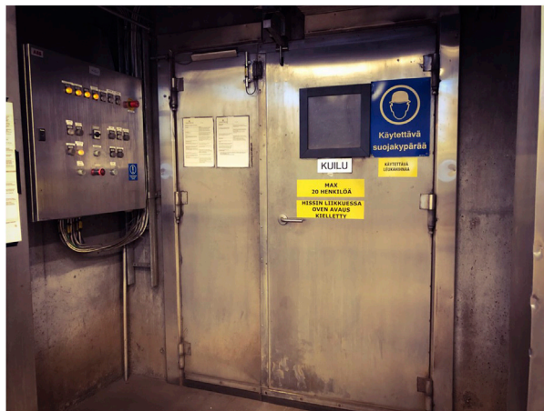
FIGURE 3 Alt Text Elevator Shaft. Access to the bottom of the mine takes less than 3 min by elevator. The journey is 1.4 km long. Picture by the second author.
