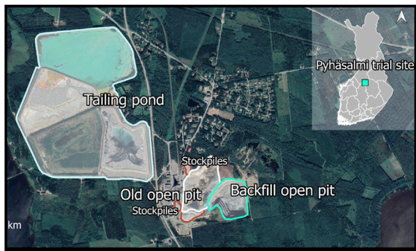
FIGURE 2 Alt Text Pyhäsalmi Mine Aerial. Callio Lab's research environment is not limited to the underground but utilizes the whole industrial area for various research purposes. Picture by second author.
