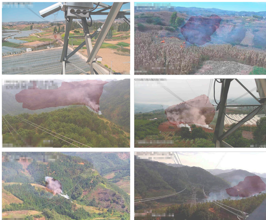
FIGURE 8 Experiments on images of electric power transmission lines. Reproduced from the Yunnan Electric Power Company, with permission from the Company.
