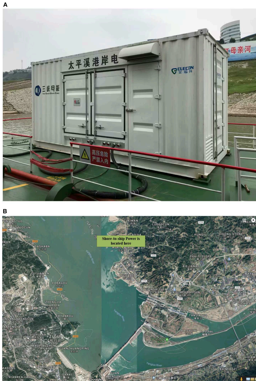
FIGURE 2 | Shore-to-ship power charging piles (China Three Gorges Power Corporation) and a map of their location beside the Yangtze River. (A) Shore-to-ship power charging piles set up by China Three Gorges Power Corporation with no cable lifting device and connection system. (B) The shore-to-ship power charging piles are located on the upper right bank of the Yangtze River Three Gorges Dam.
