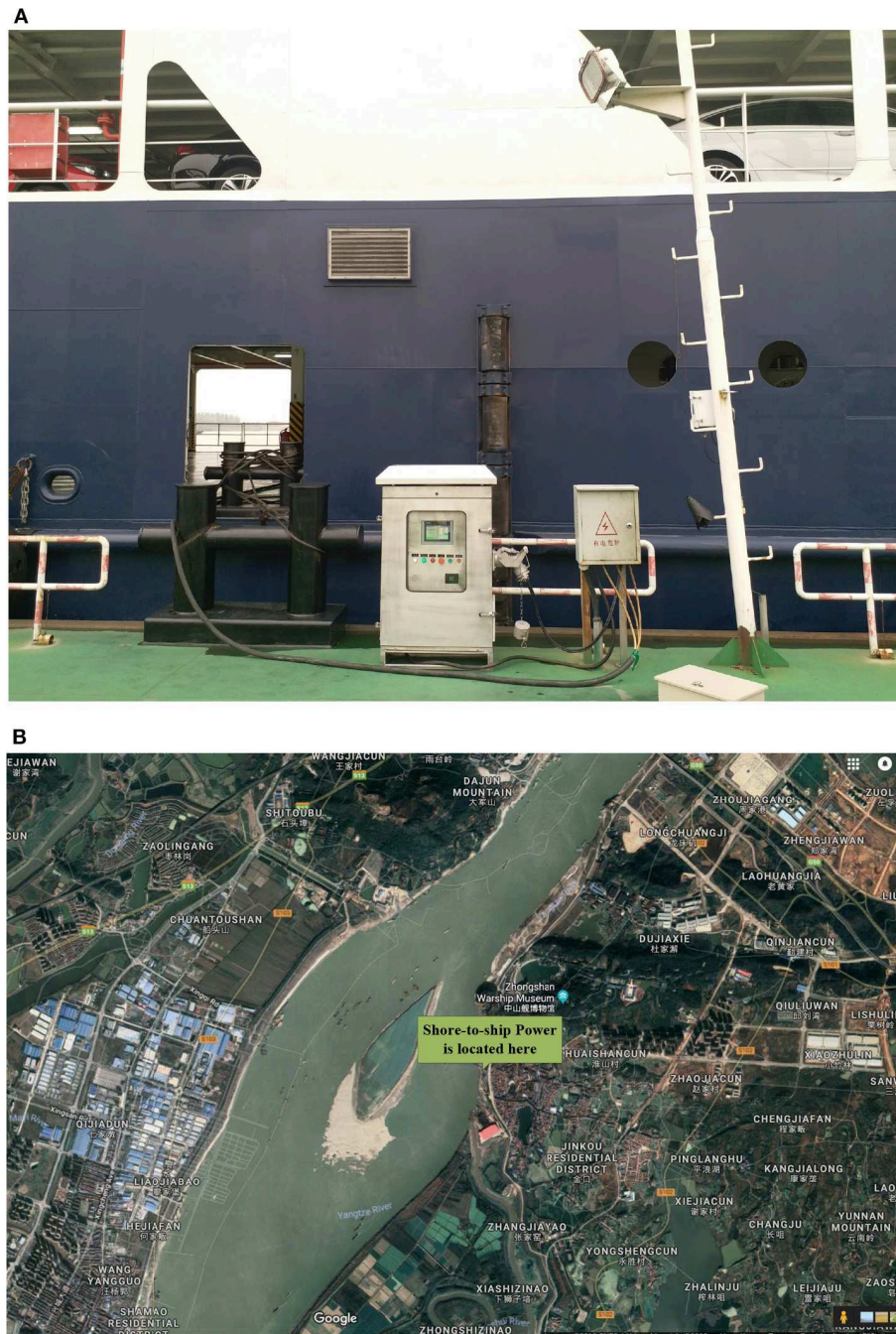
FIGURE 3 | Shore-to-ship power charging piles (Yangtze River Shipping Industry Research Center) and a map of their location beside the Yangtze River. (A) Shore-to-ship power charging piles set up by the Yangtze River Shipping Industry Research Center with no cable lifting device and connection system. (B) The shore-to-ship power charging pile was located in Jinkou Ro-Ro Terminal beside the Yangtze River, Wuhan city.
