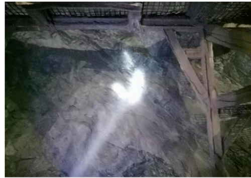
(a) ZK26+870 Tunnel Face
