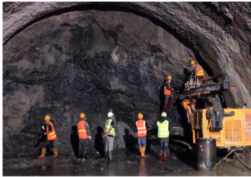
(a) ZK26+188 Tunnel Face
