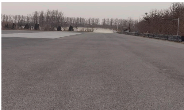
FIGURE 1 Standard test road section.
