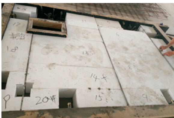
FIGURE 4 Installation of the insulation board.
