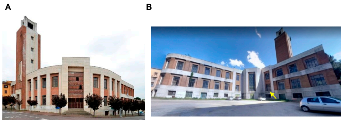
FIGURE 1 The former “Casa del Fascio”: (A) front view facing the central square; (B) rear view (the arrow indicates the location of the slab under testing).
