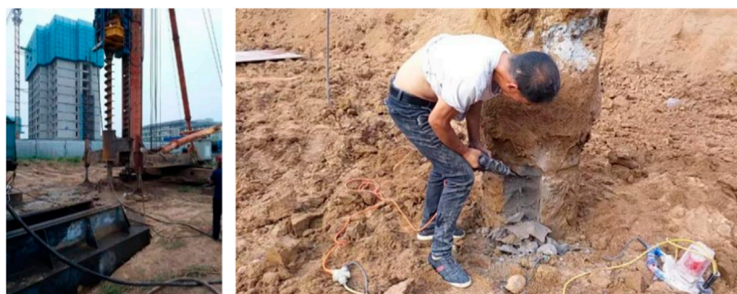
FIGURE 4 Construction photos of the in situ test.
