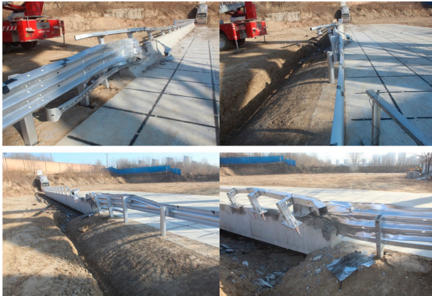
FIGURE 15 | Guardrail after the crash test.
