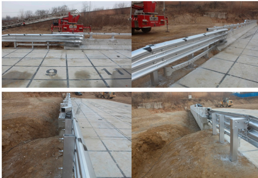
FIGURE 12 | Guardrail after the crash test.
