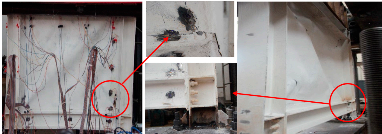
FIGURE 6 Failure phenomenon of USPSW specimen.
