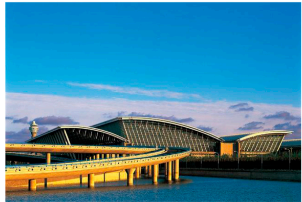
FIGURE 1 T1 terminal for Shanghai Pudong International Airport.
