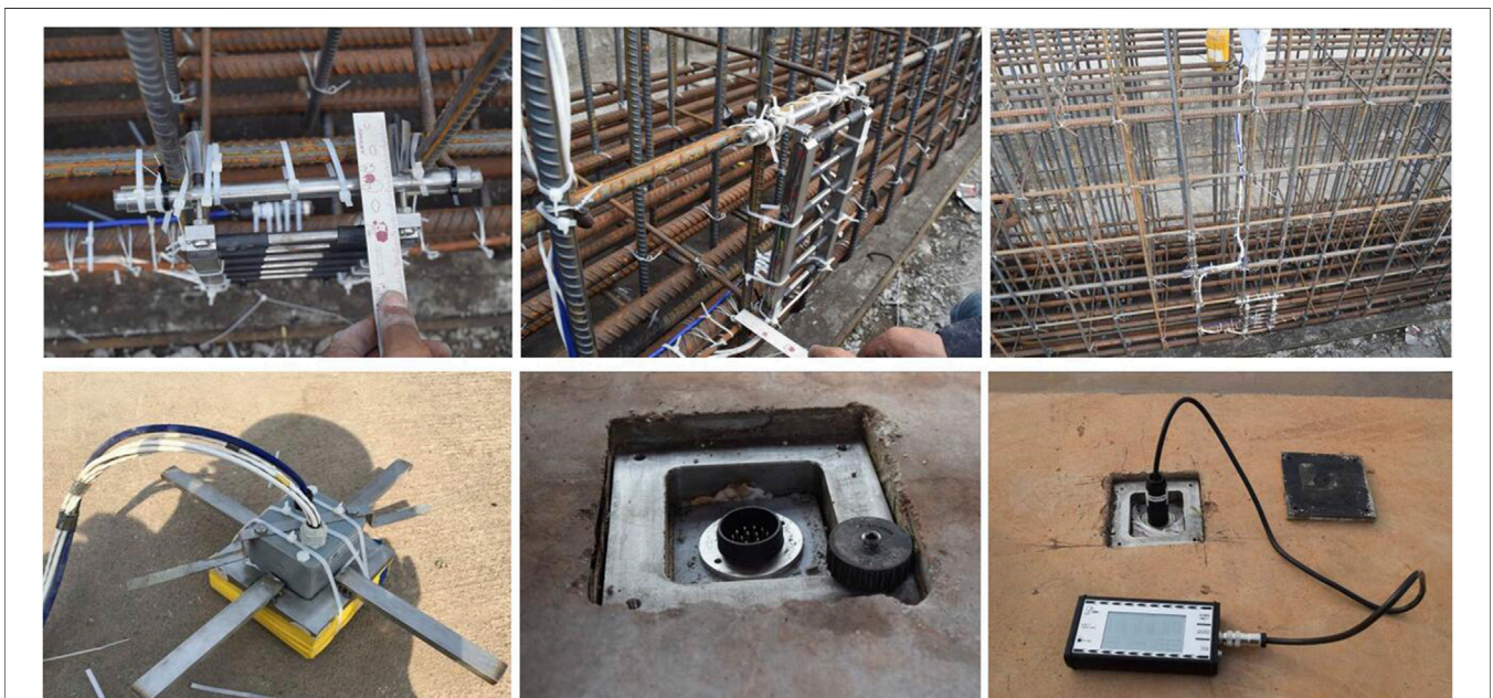
FIGURE 5 | Installation of anode-ladder sensor and field data acquisition.
