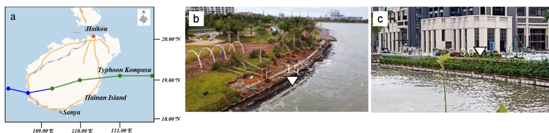
FIGURE 9 Resilience was effective during storm No.2118 “Kompasu”. (A) The typhoon path; (B) seawall facing Haikou Bay (western part of the HHCRP); (C) platform out of the embankment facing Haidian River (eastern part of the HHCRP).
