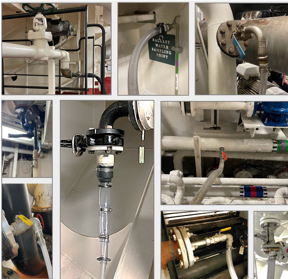
FIGURE 1 Examples of different vessels' sample port configurations that may affect sample collection.
