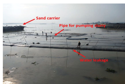
B Large geotextile mat dyke over river
