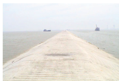
A Large geotextile mat dyke over ocean
