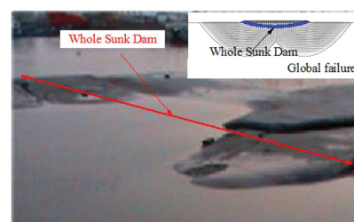
C Failure case with excessive settlement (Wei et al., 2013)
