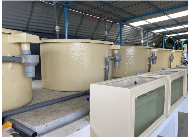
FIGURE 2 RAS units for Anthias broodstock rearing and spawning.
