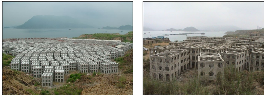
FIGURE 2 Reinforced concrete artificial reefs (3 × 3 × 5 m) laid on the seafloor in the artificial reef area of Dalajia.
