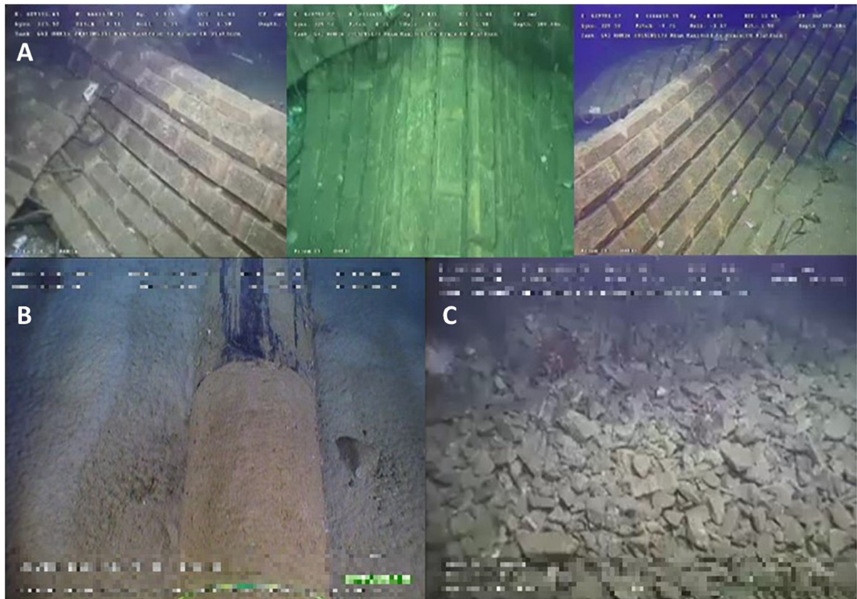
FIGURE 2 | (A) Format of ROV footage playback with three camera views (top three images left to right; port, central, and starboard) observed in synchronisation. (B) Bare pipeline and (C) rock dump.
