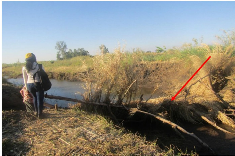
FIGURE 4 A picture showing the collapsed buffer. The red arrow points to the collapsed buffer.
