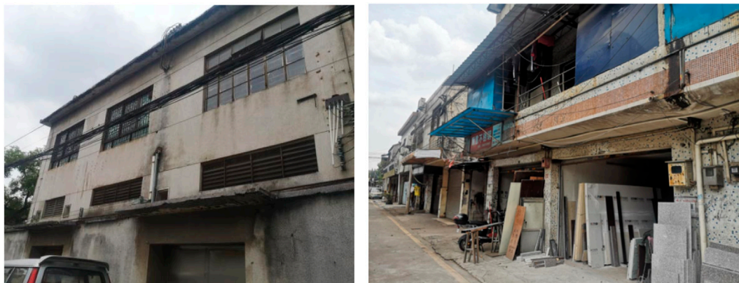
FIGURE 10 Onsite photos of Dienan Linchang Industrial Park.
