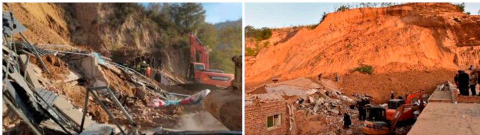
FIGURE 2 Landslides in Baota District, Yan'an City, China (In the year 2021).
