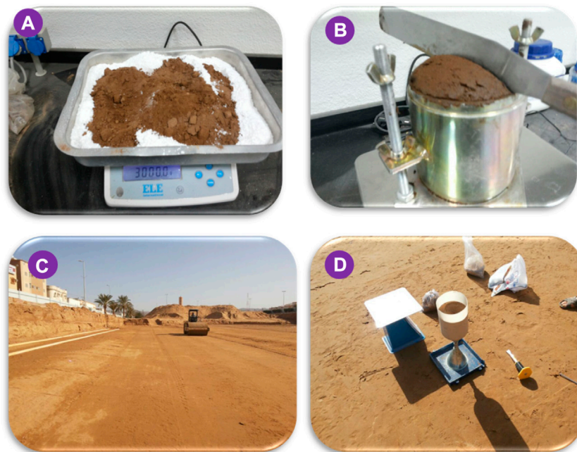
FIGURE 5 (A) and (B) Proctor compaction tests of alluvial soils with chloride in the laboratory. (C) and (D) Field density test.
