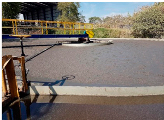
FIGURE 1 Suspended solids sample from the secondary clarifier.
