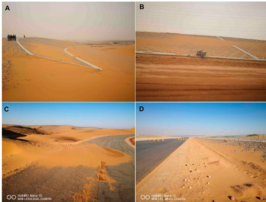
FIGURE 1 | The sand hazards on the Tengger Desert section of the Wuhai-Maqin Highway. (A) and (B) highway roadside; (C) and (D) highway subgrade.
