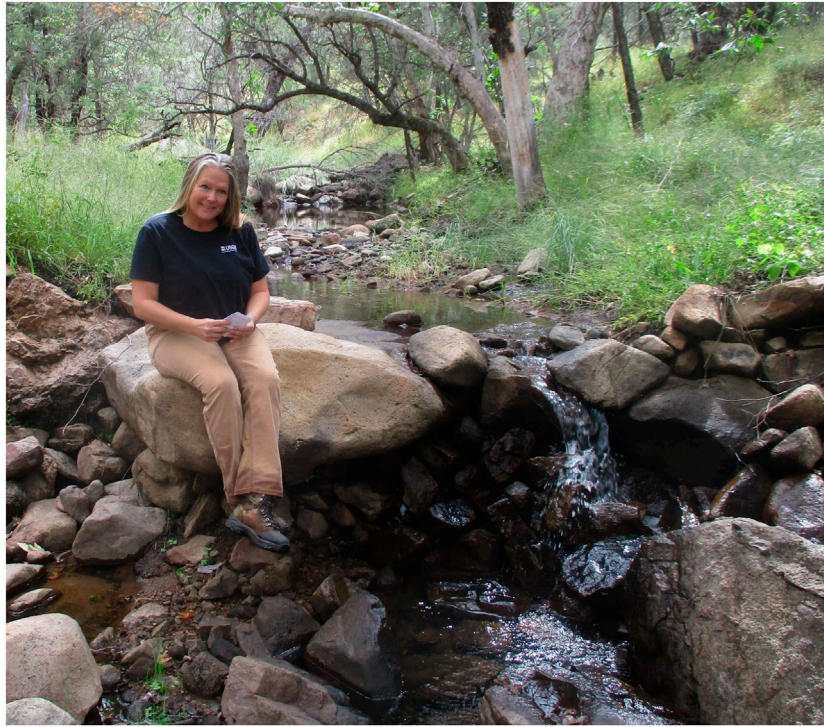
FIGURE 1 | Author sitting on a 30-year-old check dam installed at the El Coronado Ranch study area, Chiricahua Mountains, southeastern Arizona, United States (photo by Gerry Norman, Oct. 2021).
