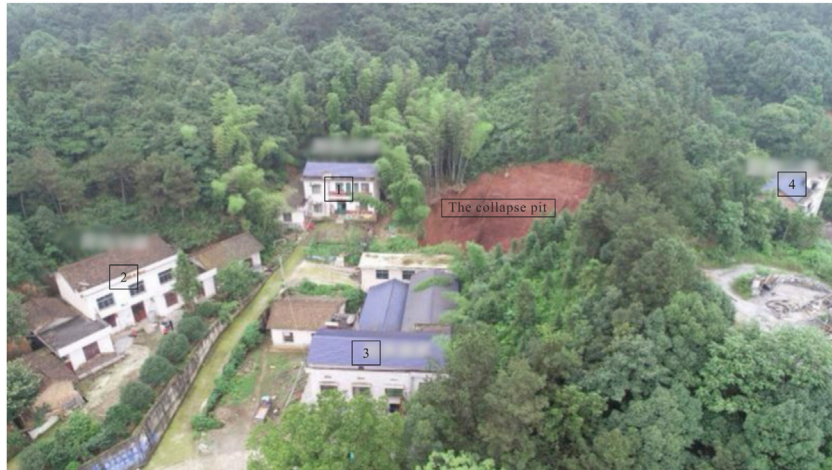
FIGURE 1 Panorama of disaster scope and affected houses.
