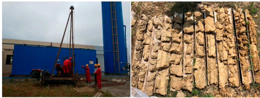
FIGURE 4 Drilling site and soil core sampling process.
