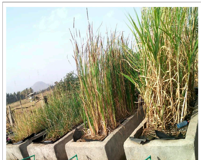
FIGURE 2 | The pilot CWUs established for the treatment of tannery wastewater.
