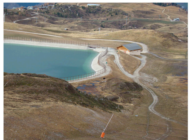
FIGURE 3 | Remnants of a wetland (2225 ma.s.l.) between a water reservoir for snowmaking and a ski run under the Roc du Diable above Belle Plagne near La Plagne Ski Resort, Savoie, France in 2011. The original wetland has been replaced by an impermeable, artificially regulated reservoir. Photo: de Jong.
